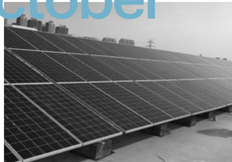
Installation of a photovoltaic system in China
